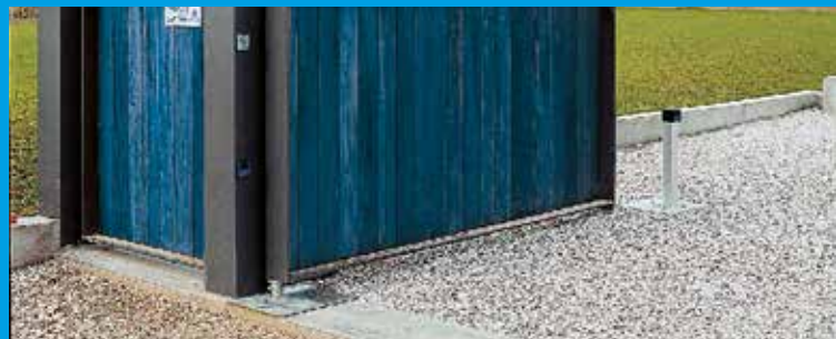
New foundation box
